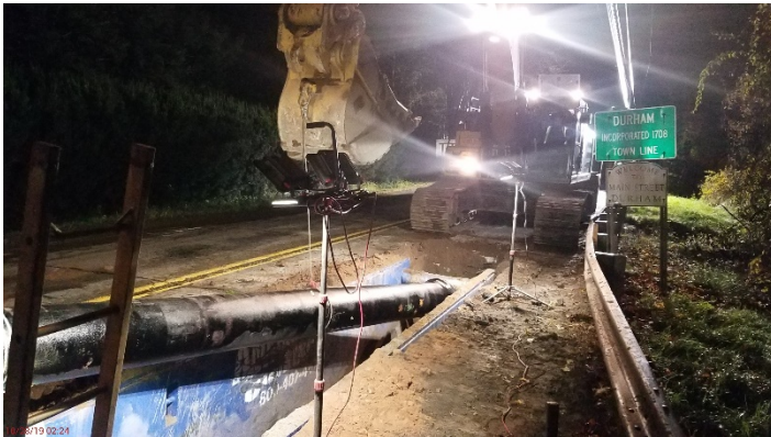
Installing 16" DIP at approximately STA # 135+00 on Main Street (Rte.17), Durham.
